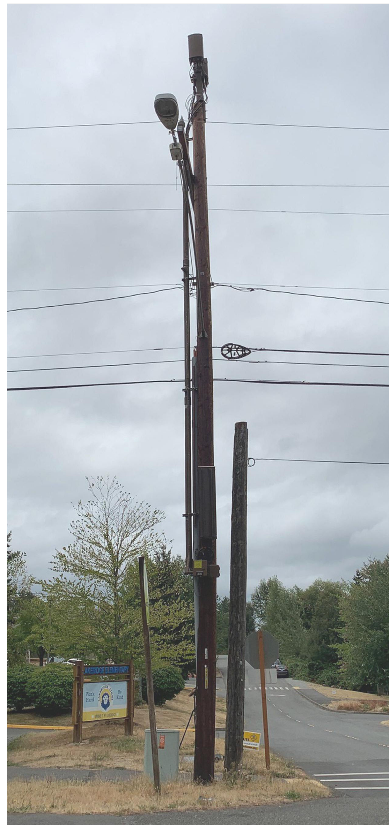
PHOTO SIMULATION - VIEW LOOKING SOUTHWEST ON SE 78TH STREET (EXISTING)
